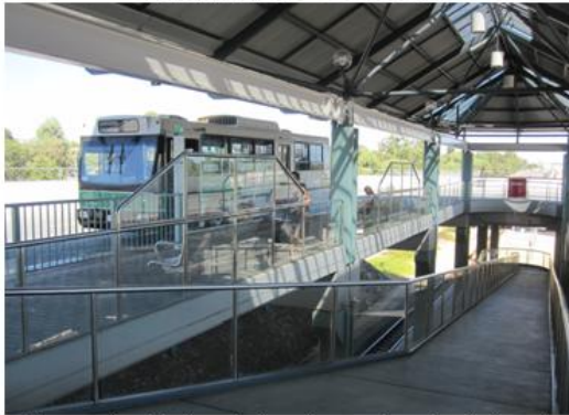
Example of a bus interchange located directly above and parallel to the station
