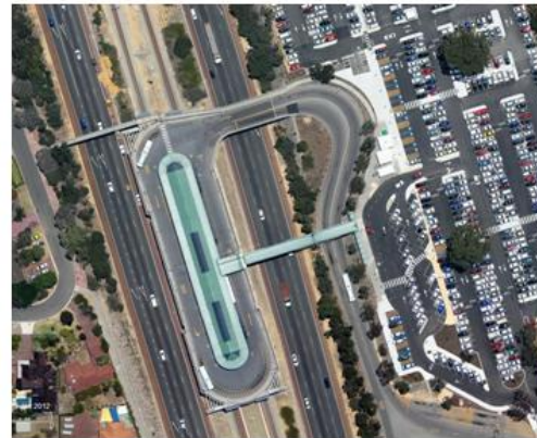
Aerial view of the station and bus interchange, bus-only overpass and adjoining Park 'n' Ride
